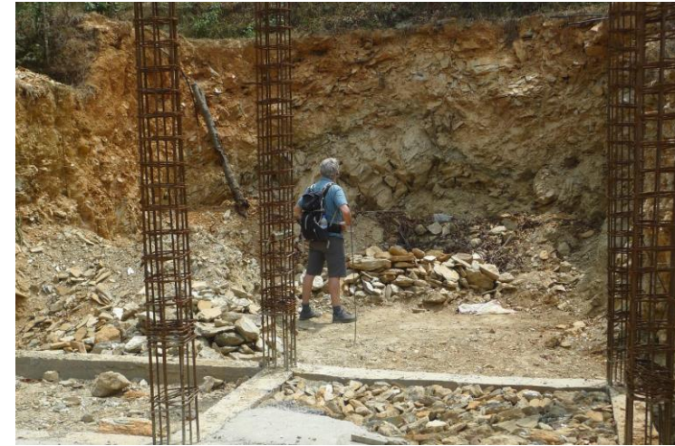
Constructing foundations in Chautara (source: A. Finlayson)
