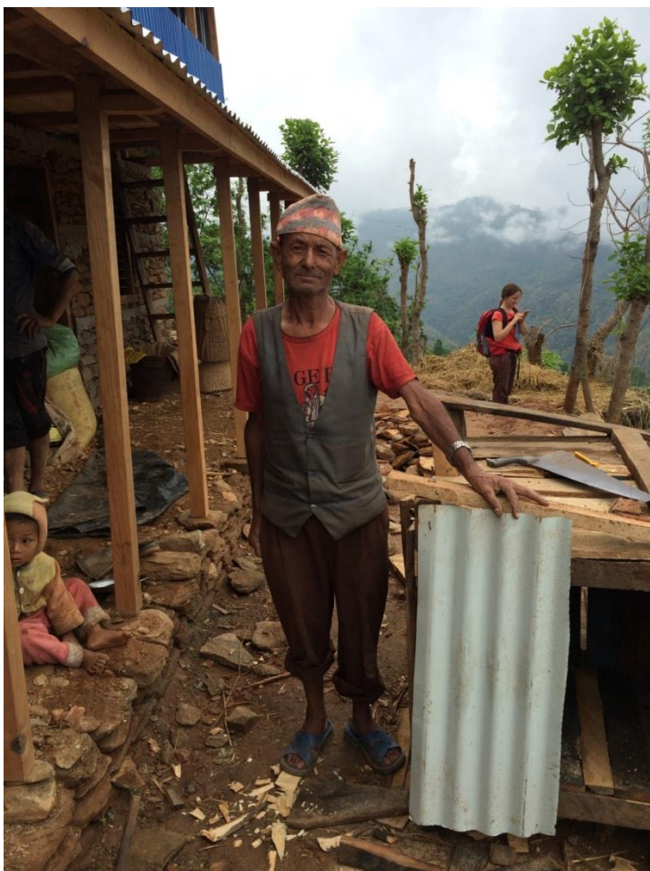
Rebuilding in Budhatum VDC, Nepal (April 2017)
